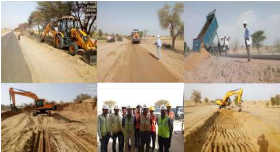
Public Works Department Road Work Kota- Sangod WIP
