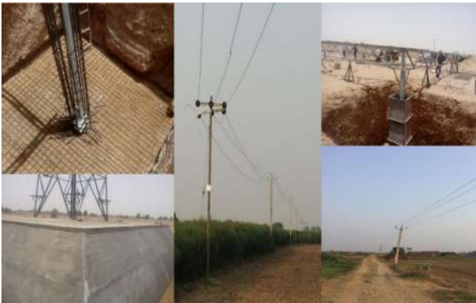
SMSA (Raj. Govt.) Building Work Alwar FY 2022-23
